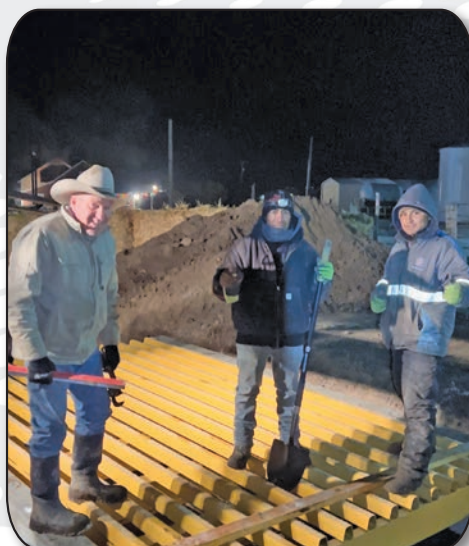
Jeff, Pedro & Frankie installing cattle guards.
