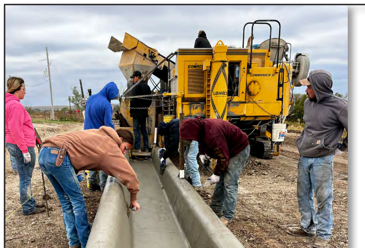
Pouring our new feed bunks
